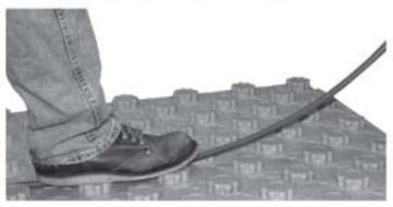
The only tip about making the PERT installation easier is that when making a turn, ensure the PERT is fully seated in the knobs before beginning or continuing a run.
