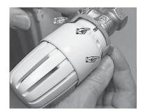
Introduce the unlocking tool up to the stop into the slot between rib ring 2 and locking sleeve 3.
