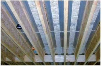
panel if screws are to be used. Staple and screws lengths should not exceed 3/4". If a pneumatic air gun is available, you could use 3/4" -16 gauge construction staples. Staples or screws should have 10 per panel, 5 per side.
