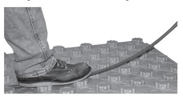
The only tip about making the PERT installation easier is that when making a turn, ensure the PERT is fully seated in the knobs before beginning or continuing a run.
